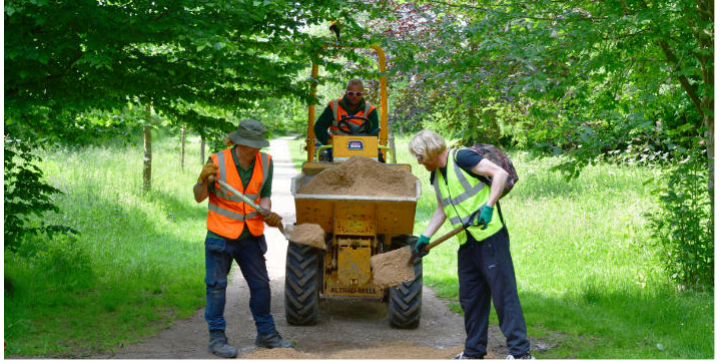
Repairing Potholes
